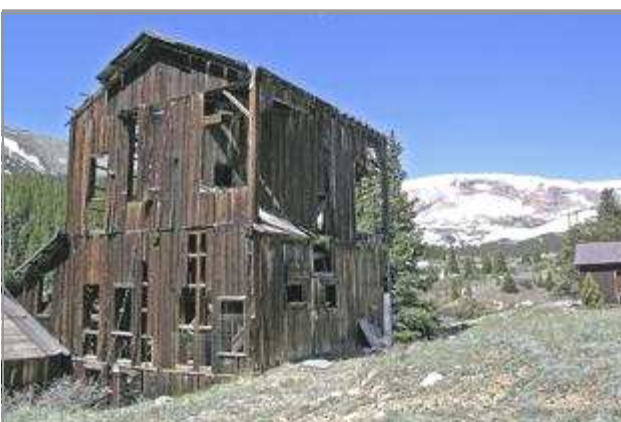
Fig. 5. Remains of the Leavick Mill on County Road 18, the Fourmile Creek Road. Photo courtesy of Park County, Colorado.
